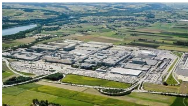
Name of building: BMW Painting Factory Country: Germany City: Dingolfing Units: VENTUS
