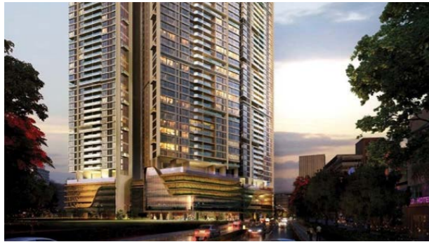
Name of building: Beaumont (Seth Creators) Country: India City: Sion Units: VENTUS
